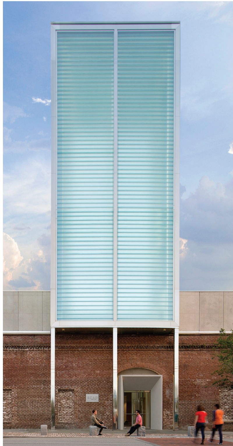
The SCAD Museum of Art's 86-foot-high steel and glass lantern atrium, and entrance. The Savannah, Georgia museum incorporates the oldest surviving antebellum railroad depot in the U.S.
